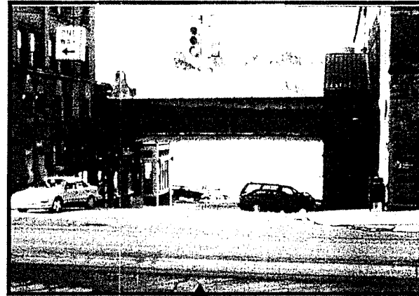
Removal of the abandoned skywalk at Isle Royale Street would open the view to the waterway and the "Mattila Square" area.
