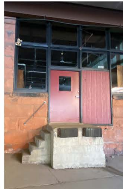
Door access for loading lower level storage and businesses
