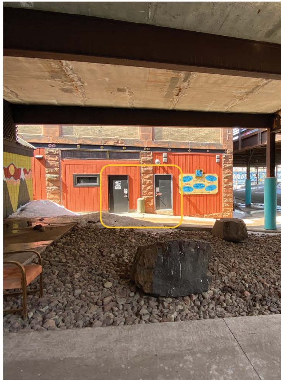
Access doors to lower level, will be preserved with new infill park.
