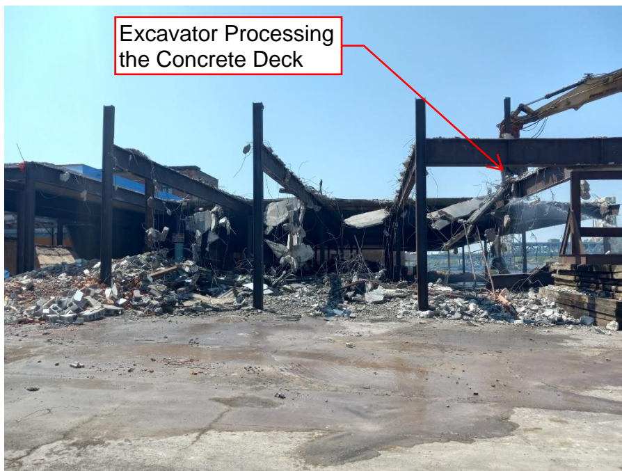
Photo of the Eastern Deck Demolition
